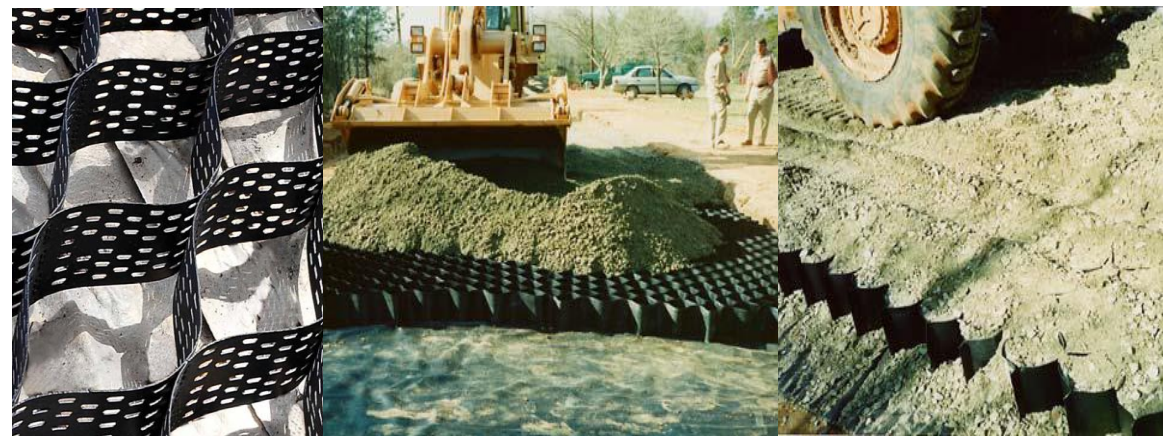
Figure 12: Increasing load bearing capacity using a Cellular Confinement System
